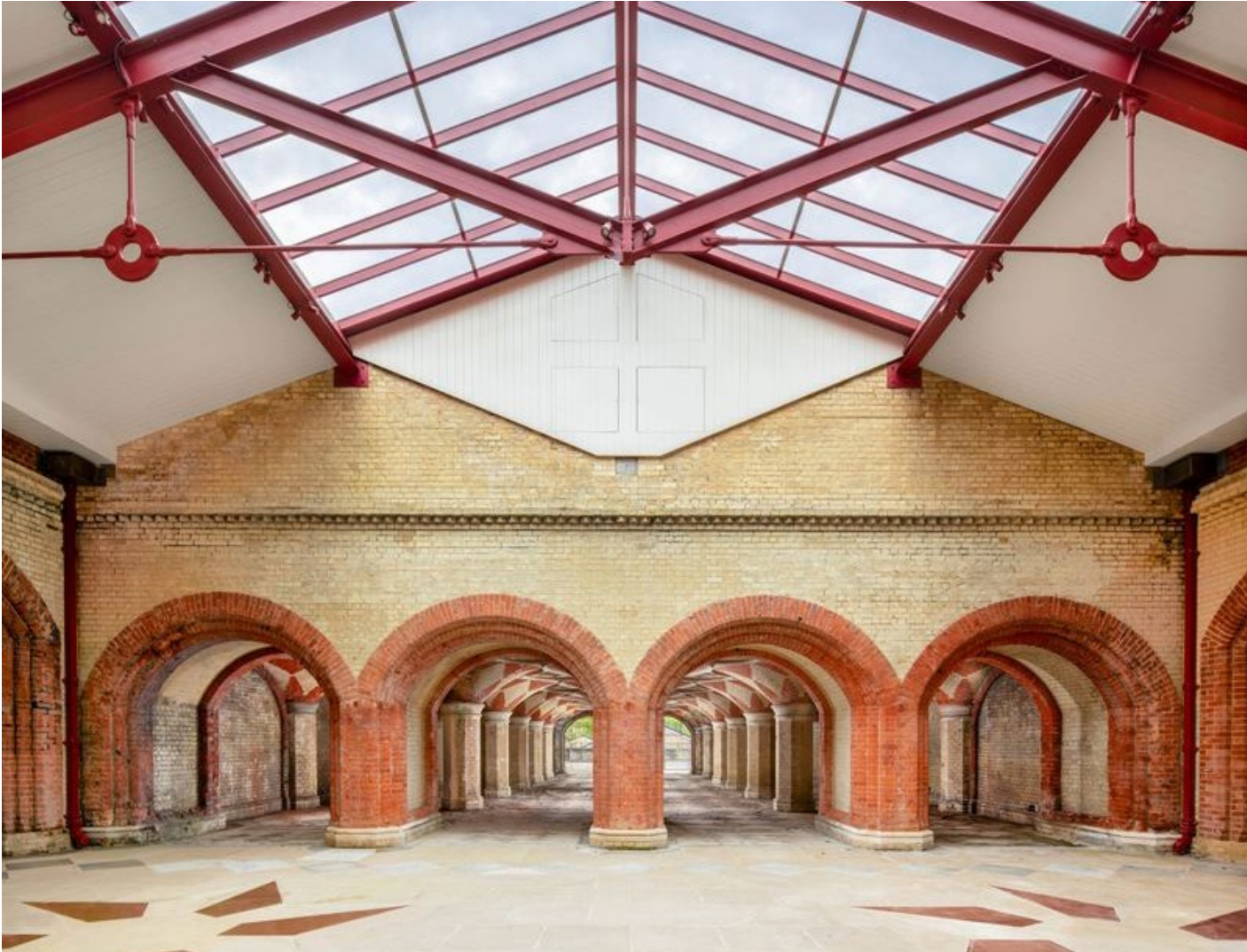
Crystal Palace High level Station Subway
