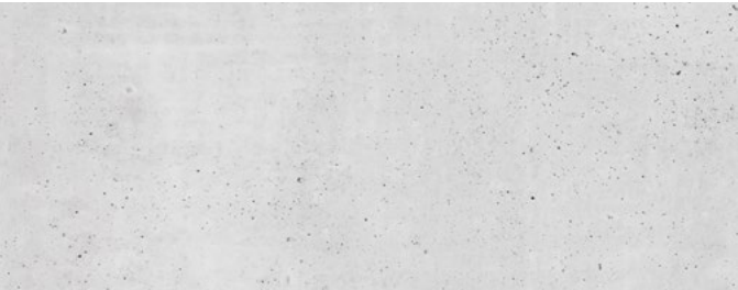
Exposed concrete to be restored (previously painted blue)
