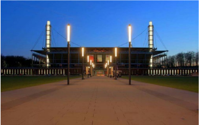
Entrance lighting at Cologne Stadium
